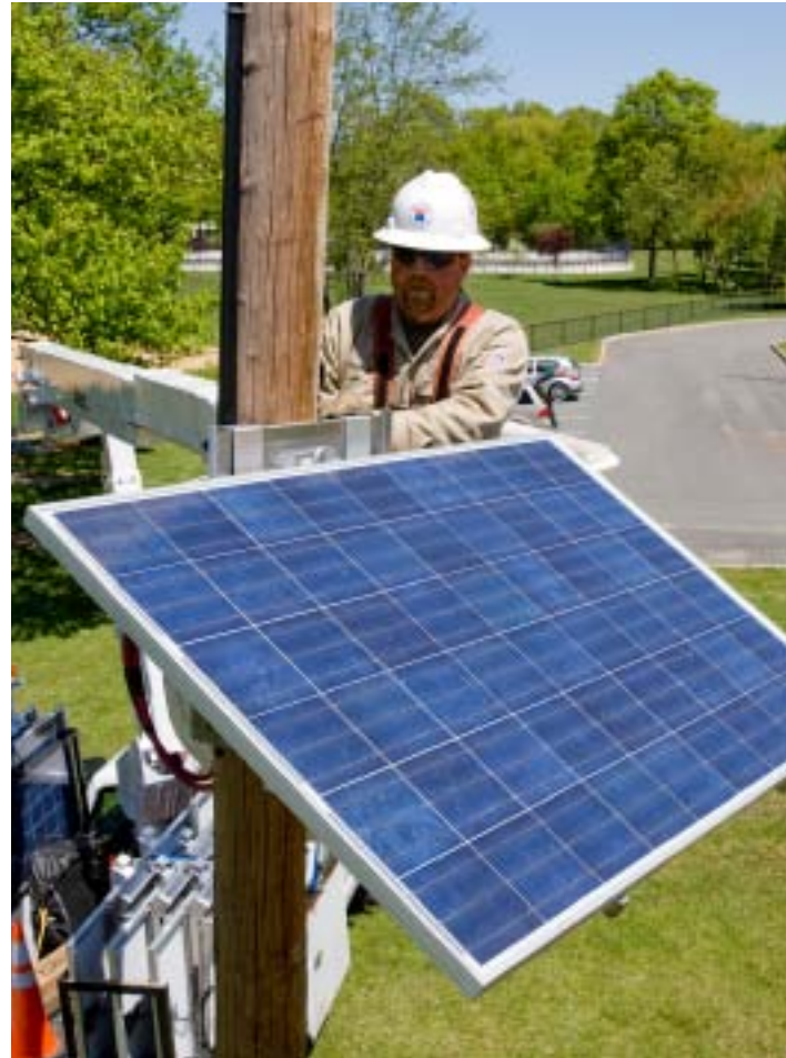
SunWave photovoltaic systems mount to streetlights and utility poles and function as a power management system connected to the smart grid.
